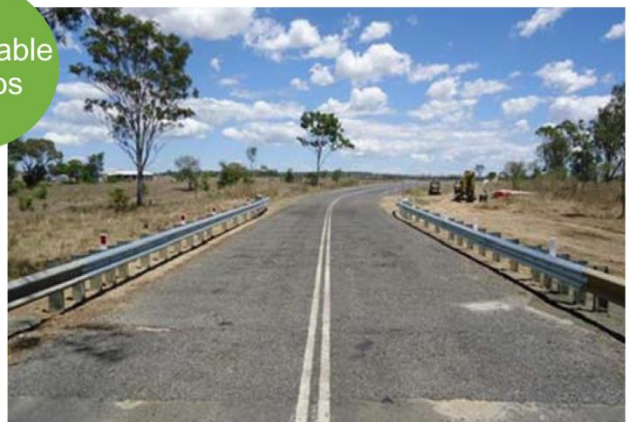
Completion of reconstruction works
