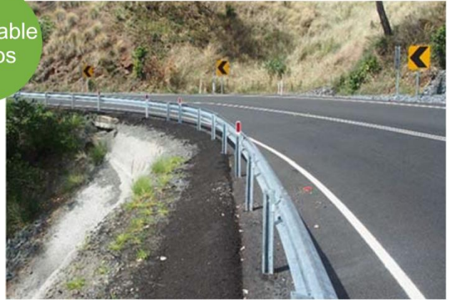
Completion of reconstruction works
